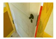
One or more interior doors do not latch. You should make adjustments or repairs as needed.
