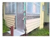
The stoop railings are not "child-safe". This means that the spacing between the balusters is wider than 4 inches. Corrections should be made to the railing construction to prevent a child from passing through the railing.
