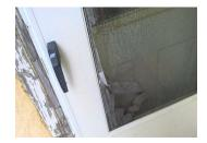
The exterior door lock is damaged or missing. This is a security concern. You should have the lock repaired or replaced. SIDE DOOR
