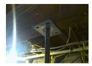
The main support is not supporting the floor joists at various areas. Recommend to have a contractor look at it for repairs.
