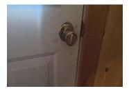
★ There is evidence of amateur workmanship. HOLLOW DOOR USED AS EXTERIOR DOOR. DOOR NEEDS REPLACING
